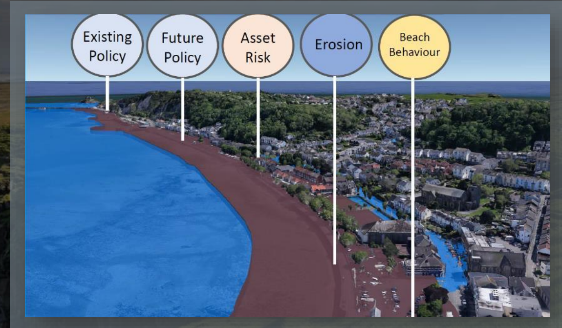
Fig.1 Key factors influencing RBM score and a demonstration of the Tidal Flood Risk Model (blue) and erosion (brown) buffers used to capture and quantify asset risks in Mumbles, Swansea.
